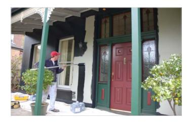
4) The side of the house is also painted with HSF 54 shielding paint and fully shielded.
