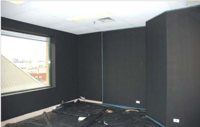
8) Now shielded, meter reading in the larger office is down to only 1.34 microwatts per metre squared.
