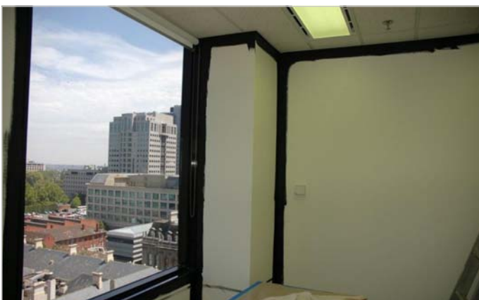
5) Shielding paint being applied.
