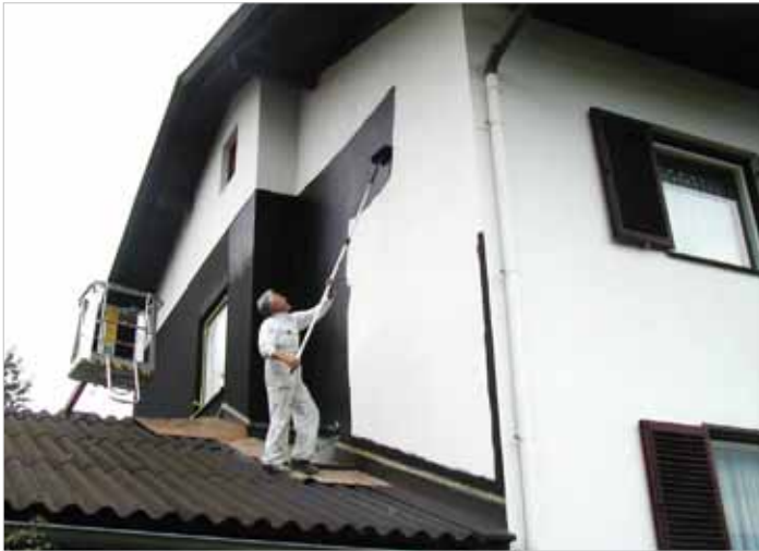
3) Grounding of the shielding paint.
