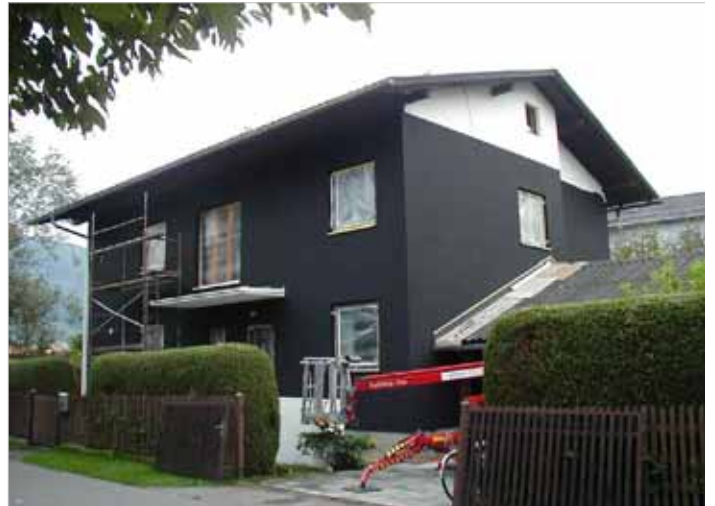
4) Application of the top coat.
