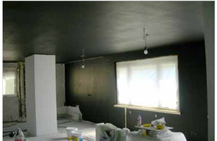
4) They used shielding paint HSF54.
