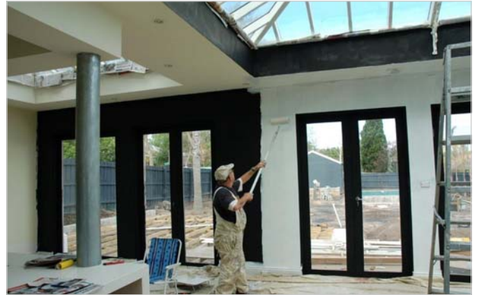
8) Two quick easy coats of acrylic wall paint cover the black shielding paint.
