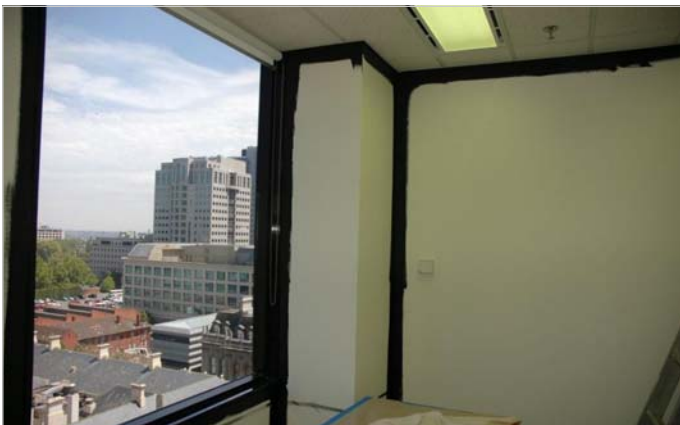
5) Shielding paint being applied.
